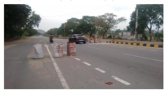
To prevent collision of vehicles coming in from Lane Crossing and vehicles travelling on main lane, barricades are being erected. By which NHAI is creating a situation where vehicles have no other option but to reduce the speed in that particular place. Even after spending so much money, time, and effort and converting Two lane Two way highways to Four Lane Two Way Highways, if free traffic flow is not possible, are the methods implemented by NHAI beneficial?
